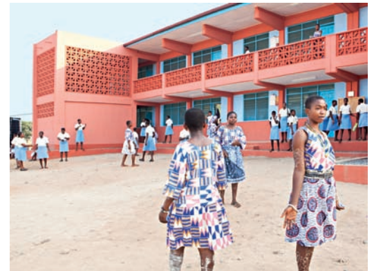
1. Bauabschnitt - Schlaftrakt | 1st construction phase - dormitory
